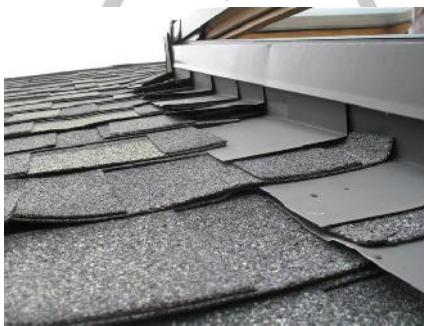
Lifting skylight flashing
